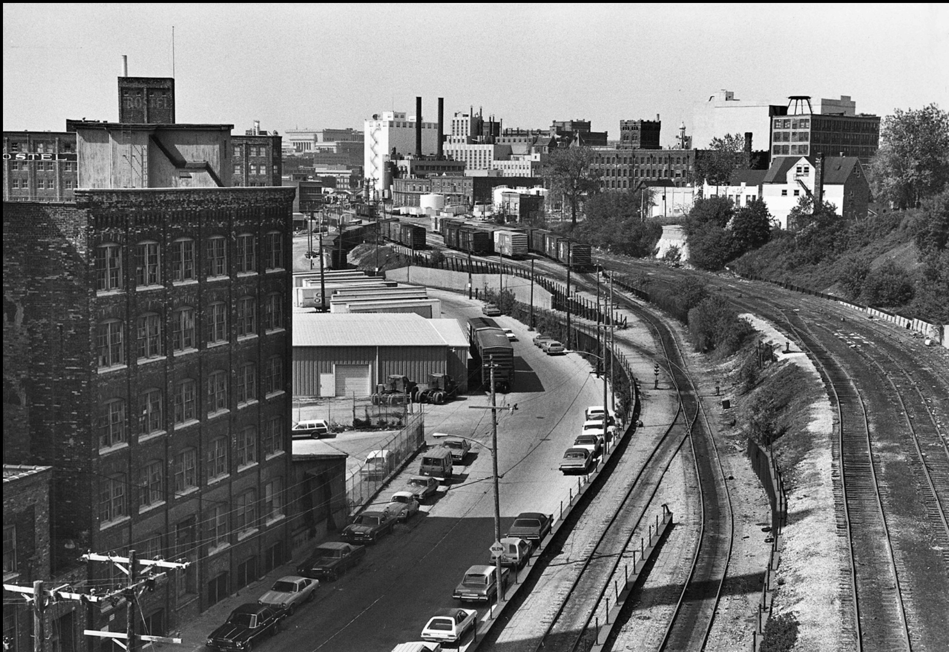
The Milwaukee Road's Beer Line in the mid-1970s, with Schlitz and Mayer Boot & Shoe Company in the distance, and the Trostel Tannery on the left. Mike Schafer photo
