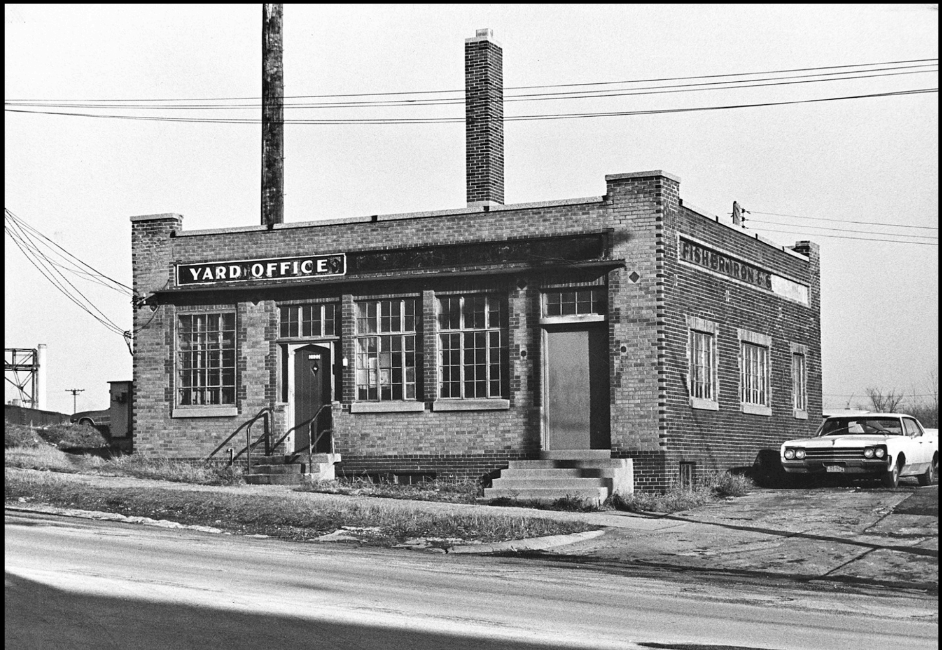
Milwaukee Road's Humboldt Yard office, December 1974.
